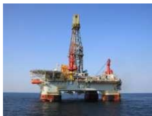
Offshore drilling platform
