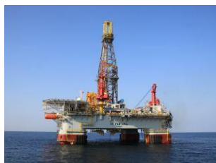
Offshore drilling platform
